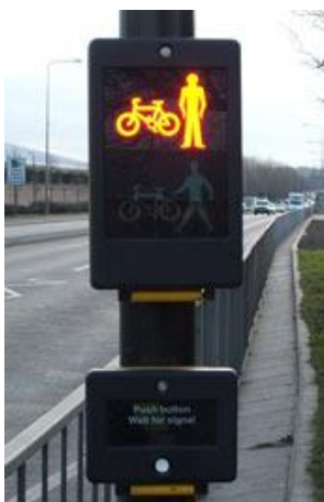
Toucans are used in the UK to allow cyclists to cross with pedestrians. They use on-crossing detectors, like puffins, and cost about the same as puffins to install. Photo via newcastle.gov.uk.
