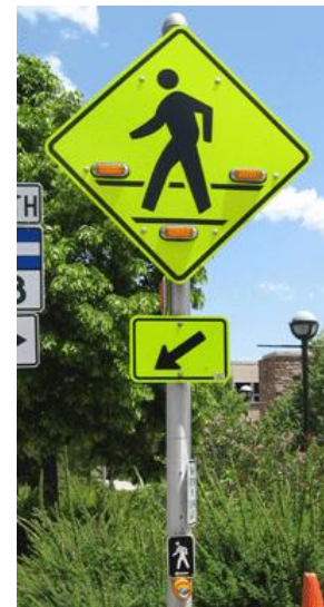
Boulder zebra crossings are enhanced with pelican push-button crossing technology. And pedestrian actuated lights on signs by crosswalks alert motorists when people are crossing. Photo via BoulderColorado.gov.
