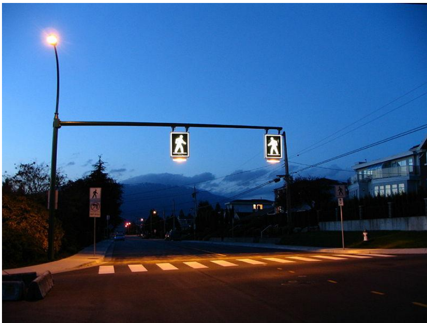
A zebra crosswalk in Burnaby, BC, Canada is enhanced with lit overhead signs. Photo via wikimedia.org.
