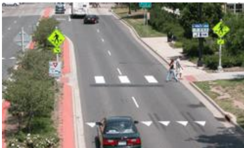
In Boulder, Colorado, cars are required to stop before the "yield line" to ensure they remain a safe distance from pedestrians at the zebra crossing. Photo via BoulderColorado.gov
